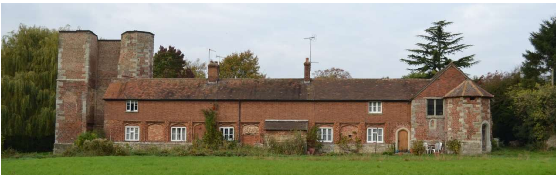
Figure 3: The view from the South after the first phase of repairs in 2016
